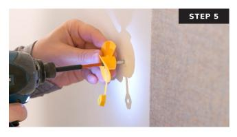
Screw Rotofast Standard Anchor to wall at marked location. Make sure the anchor spins on the shaft of the screw but does not wobble.
