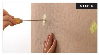
Place panel at marked location and use scratch awl to penetrate panel and mark substrate for anchor locations.
