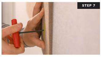
Insert the installation tool through hole in painters tape. Feel and hear the installation tool engage with the insert. Turn the Rotofast anchor counter-clockwise (left) while firmly pushing the panel toward the wall.
