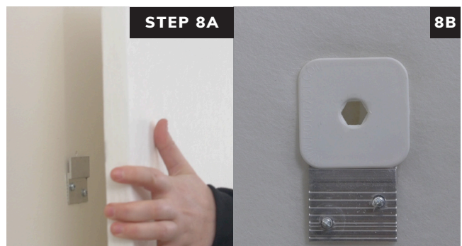
Line up the panel. Slide down until you feel the flange contact the top of the Z CLIP. Push in on the panel and slide it down to engage the Z CLIPS. Make sure all clips are engaged to complete installation.
