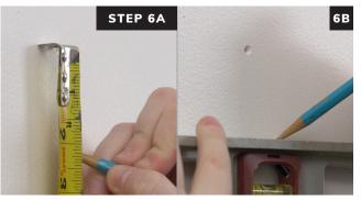
Measure down 2" from each mark. Use a level to make a short line at this location.
