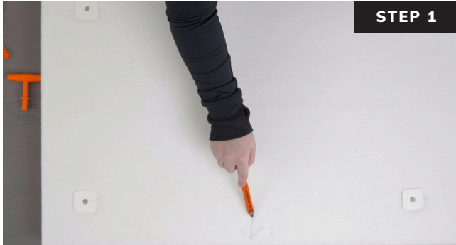
Measure and mark the location where panel will be placed and mark the orientation on the back of the panel.
