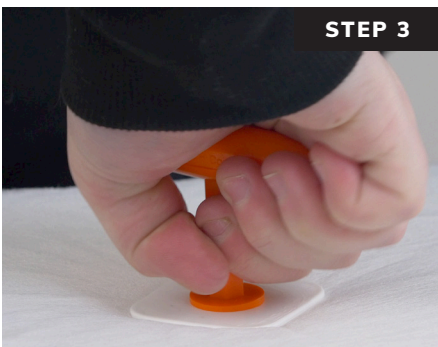
Screw Rotofast Snap-On Anchors into back of the panel using the Rotofast driver tool. Do not over-tighten.
