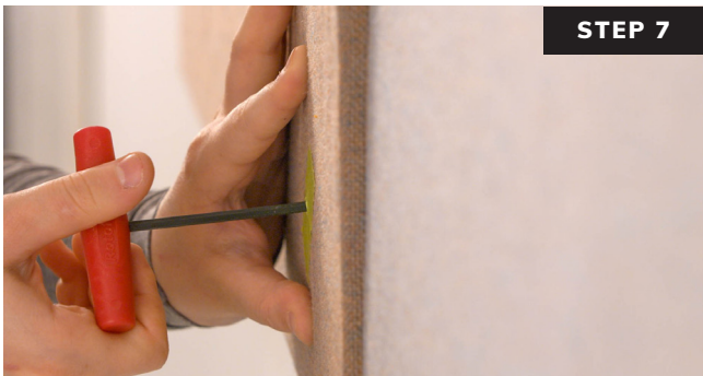
Insert the installation tool through hole in painters tape. Feel and hear the installation tool engage with the insert. Turn the Rotofast anchor counter-clockwise (left) while firmly pushing the panel toward the wall.
