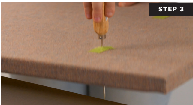
Push the scratch awl through the panel at the marked locations, keeping the scratch awl as straight as possible.
