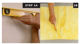
Measure and mark the location where panel will be placed. Also mark the orientation on the back of the panel.
