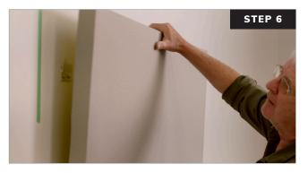
Remove the marking plugs. Slide the panel down, engaging the EZ Clips with the Z bars.
