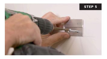
Install a Z bar at each level line, centered on the mark.
