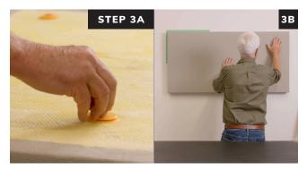
Insert reusable marking plugs into the EZ Clips. Push panel against wall to mark EZ Clip locations.
