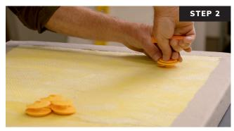
Screw Rotofast EZ Clips into back of the panel using the Rotofast driver tool. Do not over-tighten. Make sure the flange is parellel to the back of the panel.
